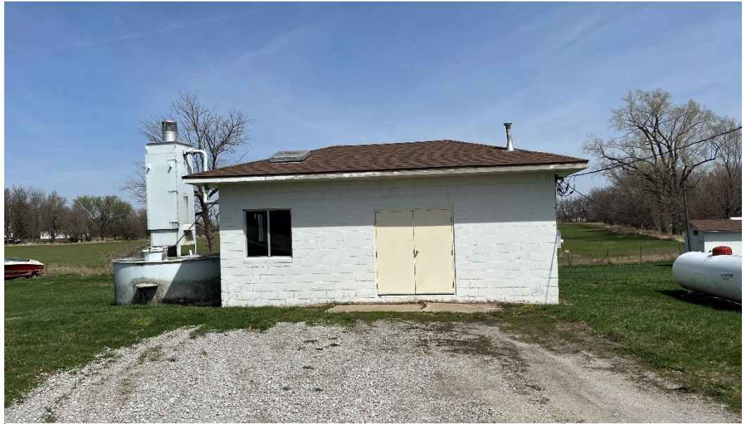
Figure 7 – City of Randolph Water Treatment Plant
