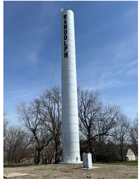
Figure 10 - City of Randolph Standpipe
