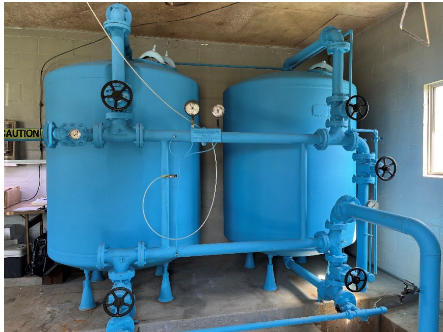
Figure 8 - City of Randolph Pressure Filters
