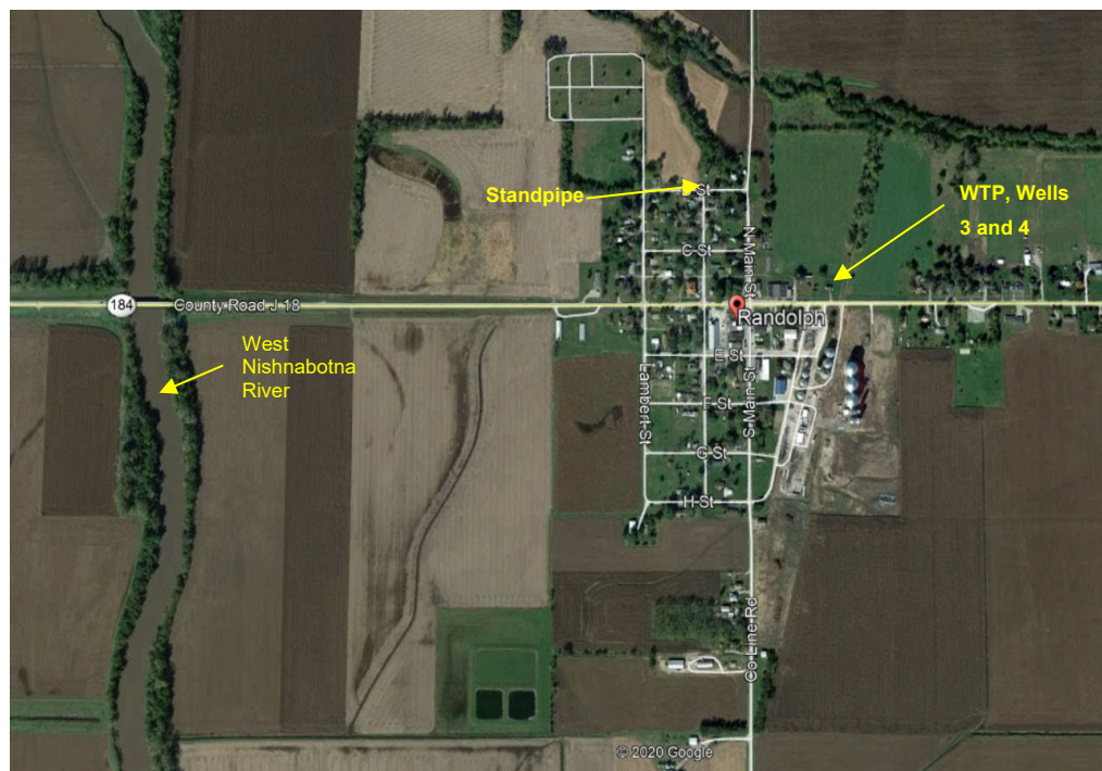
Figure 1 - Aerial Photo of Randolph
